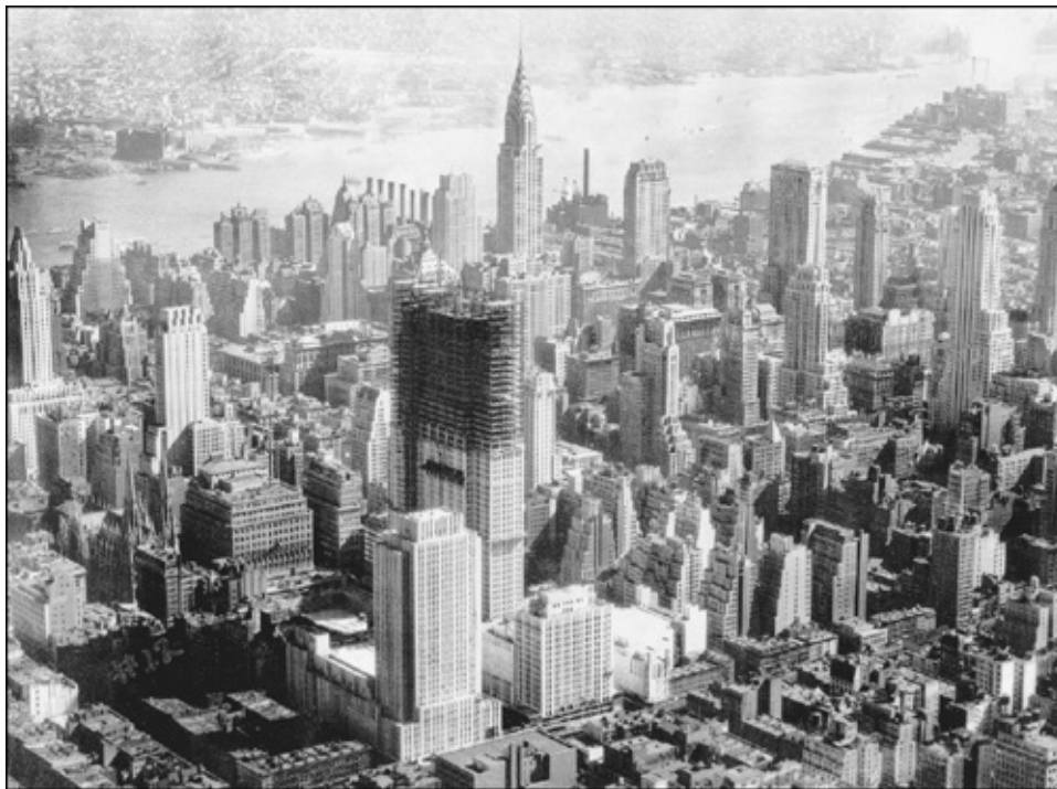
Rockefeller Center under construction. The Center was Father's great gamble with the fortune Grandfather had entrusted to him. This 1932 photo shows the RCA Building nearing completion,
