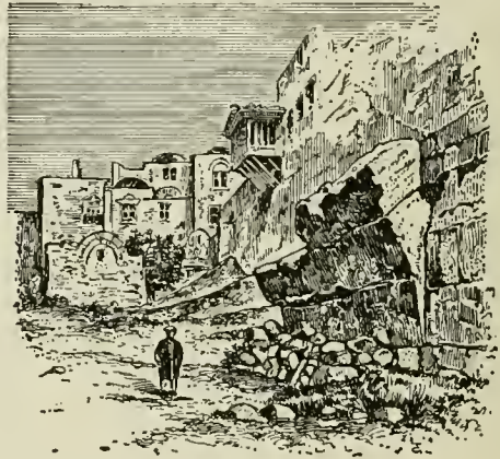
Remains of Arch of Bridge.
