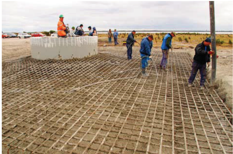
Gravitationsfundament. Foto: Gunnar Britse, WindPower Photo.
